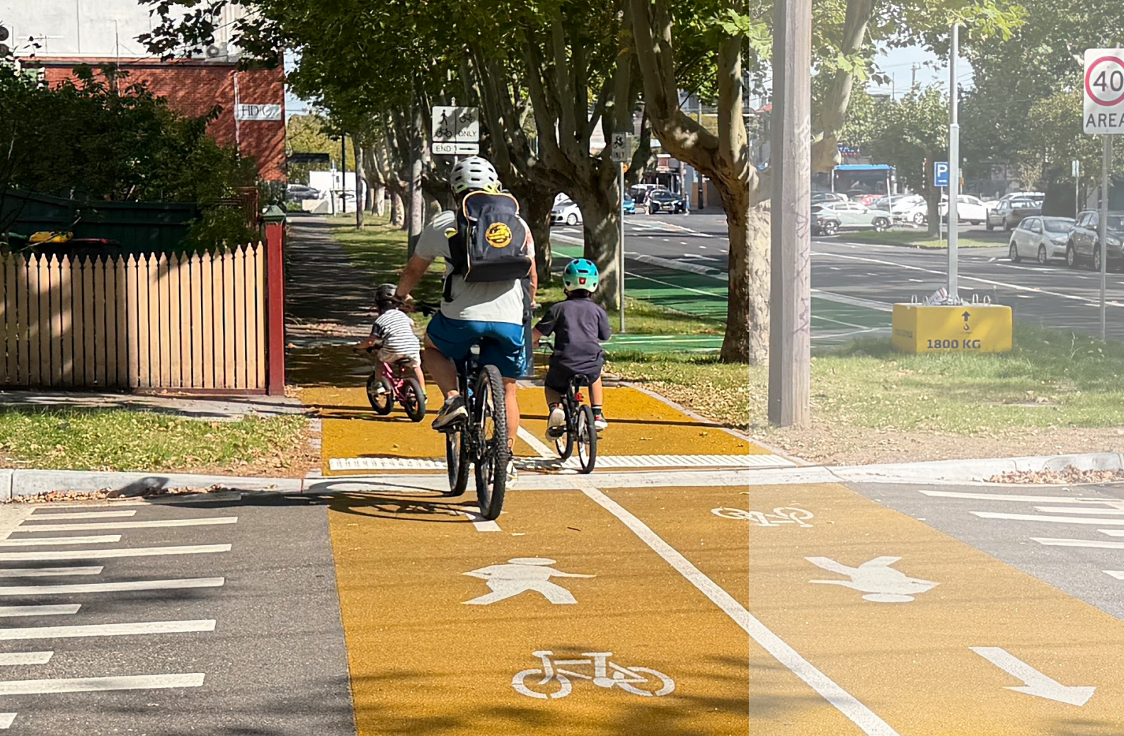
Oakleigh's new two-way cycleway on Atkinson Street.
